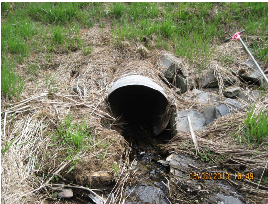
Photo 4. View of Stream A culvert
