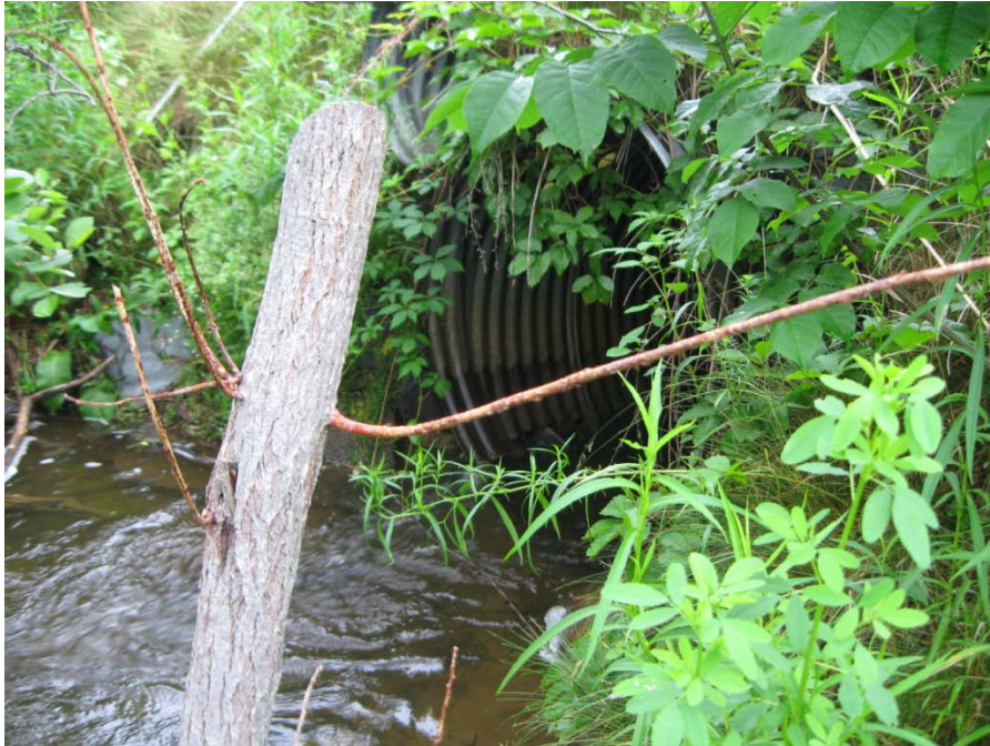
Photo 7. Trafton Brook culvert crossing
